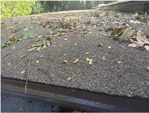
923-2 Rolled Roofing Carport/Enclosed Porch
