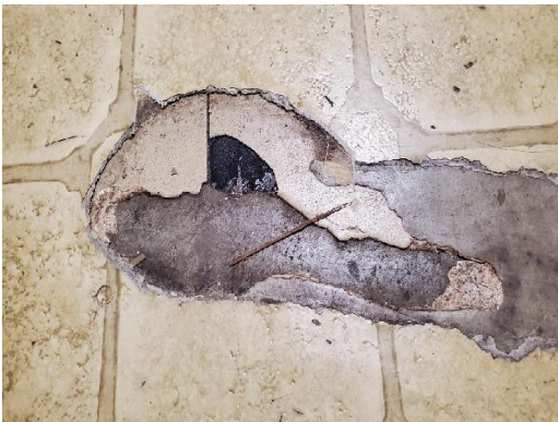
923-4 9"x9" Floor Tile (2% Chrysotile) Mastic Interior Kitchen (approx. 150 sq. ft.)
