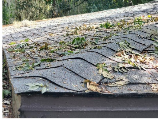
923-1 Asphalt Shingle/Tar Typical Exterior Roof
